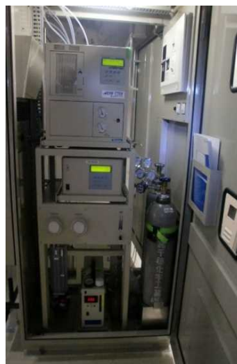
Inside of the cubicle
