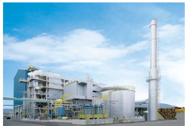
Wood Waste Fired Boiler Plant Hiroshima Prefecture, Japan 5,000 kW
