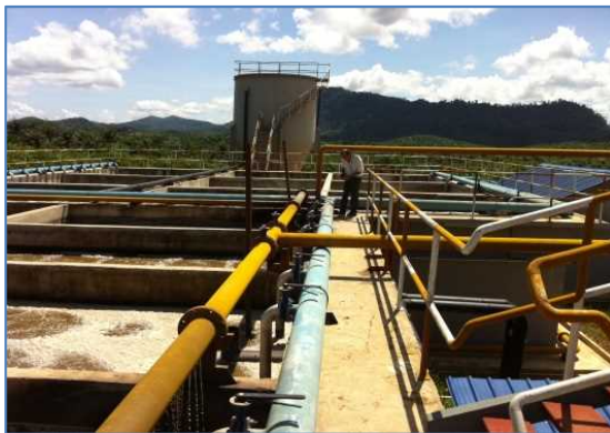
Malaysia SD Palm Oil factory wastewater treatment system , BOD20 Plant. Influent volume 960m 3 /D by AeratorS1 72sets
