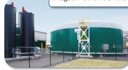
Convert biogas to electricity by utilizing microorganism decomposition process from various organic waste.
