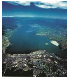
Planning on water quality preservation in Nagaragawa Estuary Barrage
