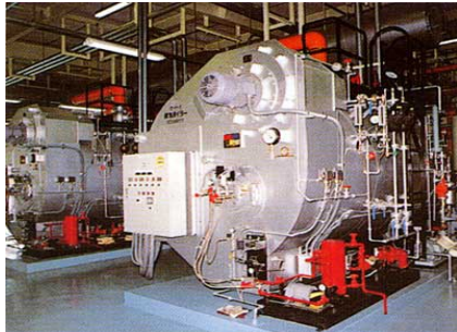
Conventional flue and smoke tube boiler
