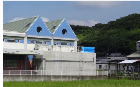
Wastewater treatment system (Industry)
