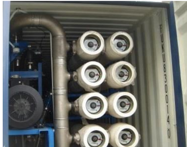
RO membrane module mounted on purification system
