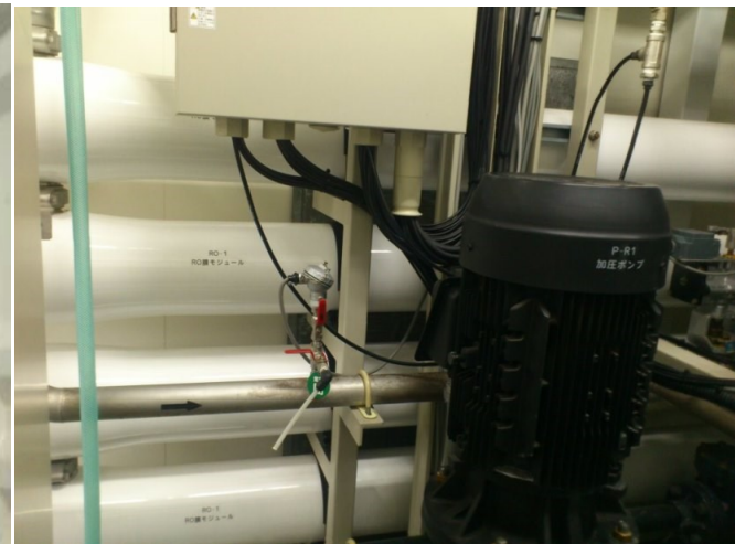
RO membrane module mounted on purification system
