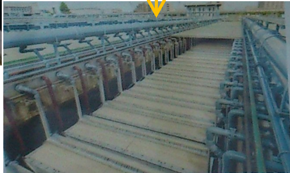
Installation of MBR at sewage treatment plant
